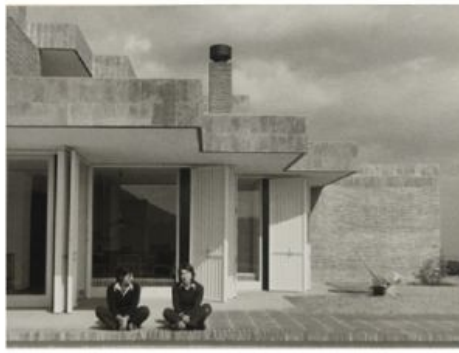
Photographs taken at Casa Coderch, Sant Feliu de Codines. Architect: José Antonio Coderch
